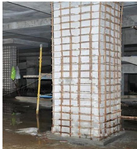
Figure 7. RC Jacketing of Columns Being Executed On Site
