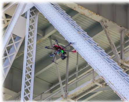
Figure 7: Bridge Inspection using UAS (Gold Star Memorial Bridge, Connecticut)
