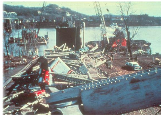
Figure 3: Collapse of the Silver Bridge
