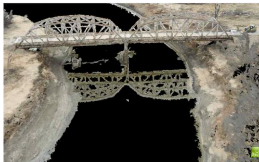
Figure 7: Bridge Inspection using UAS (Gold Star Memorial Bridge, Connecticut)
