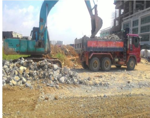
Figure 4: Concrete Waste Transported to Lorry
