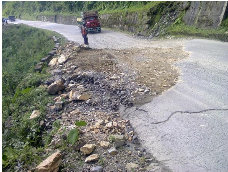
Figure 1 : Road section in Sorchen showing the sinking profile
